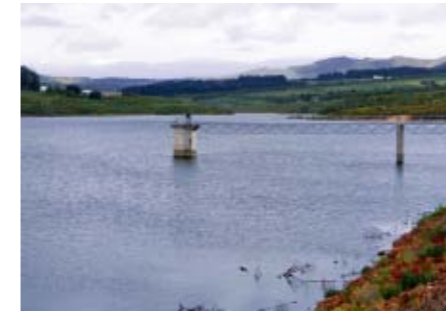
As part of water management strategies, water users are allowed to develop water infrastructures such as dams for irrigation.
