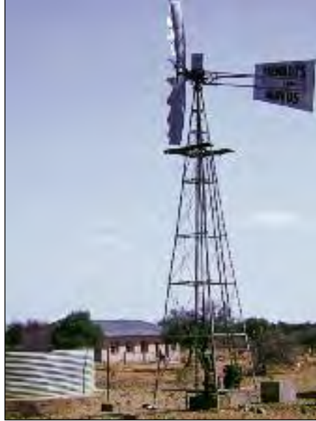
Windpump and borehole installation
