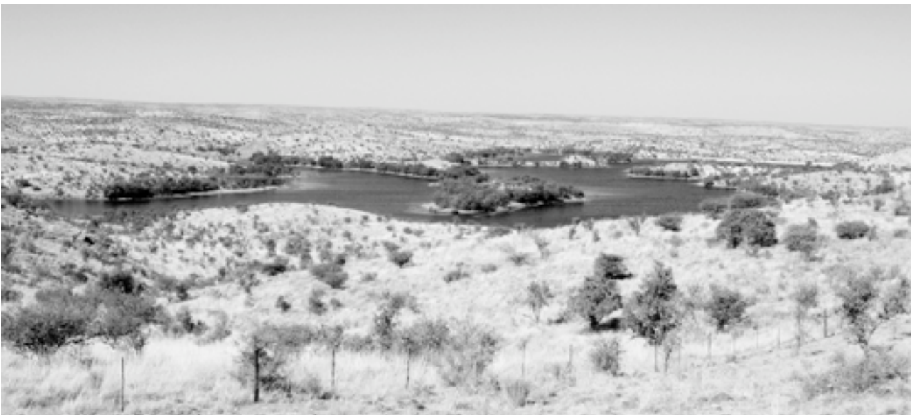
Photo 4. The Friedenau Dam close to windhoek.
